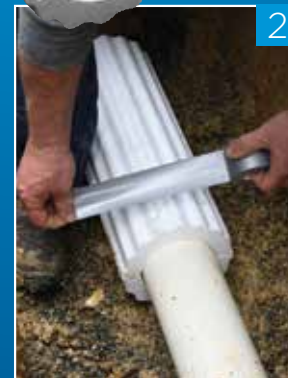
2. Fit two halves together, secure first end with duct tape
