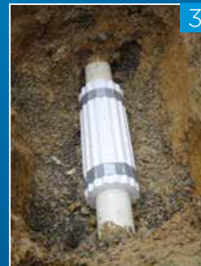
3. Secure other end with duct tape. Job completed.
