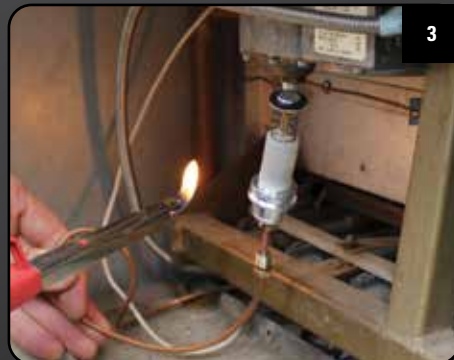
3 Light the pilot using the normal method for the appliance.
