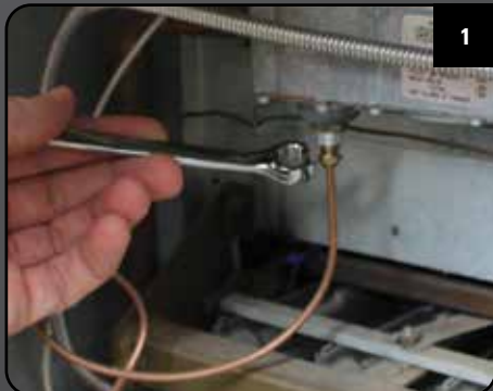
1 Unscrew the existing thermocouple from the control unit of the appliance.
