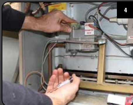
4 Whilst continuing to hold down the button on the appliance for 20 seconds, depress the spring on the testing device at the same time.
