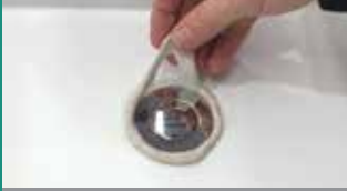
3. Remove excess compound
