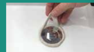
3. Remove excess compound
