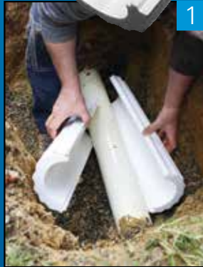
1. Take 2 pieces of Styrolag and place around pipe
