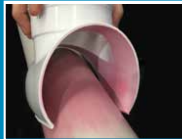
1. Apply Priming Fluid
