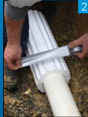
2. Fit two halves together, secure first end with duct tape
