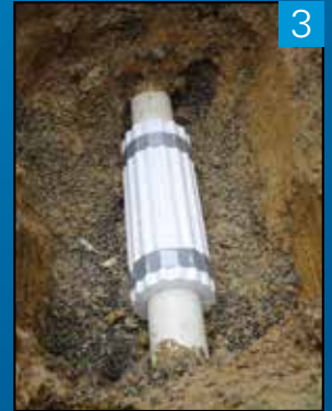
3. Secure other end with duct tape. Job completed.
