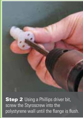
Step 1 Items required - Styroscrew anchors, suitable 8g screw, Phillips driver bit, cordless drill.
